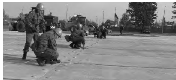
Fig. 2. Method of connecting of mat segments
